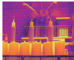
Electric routine inspection
